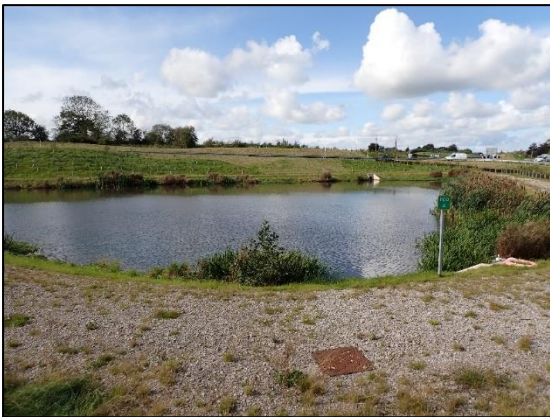
The treatment pond for runoff from the Bypass
